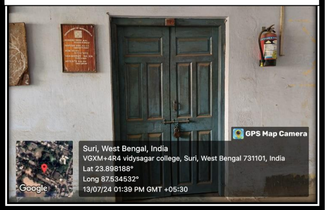
Fire Extinguisher Facility Math Department
